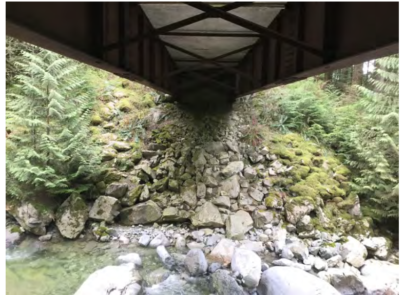
Left Bank Abutment when facing downstream
