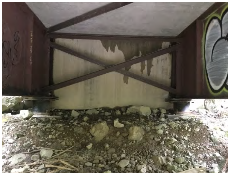
Left Bank Abutment when facing downstream
