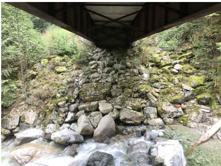
Right Bank Abutment when facing downstream
