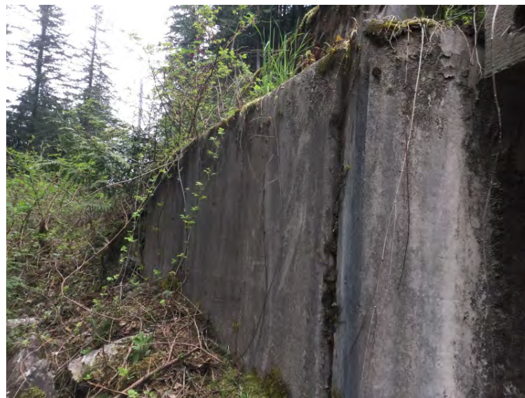
Concrete wingwall only at downstream locations
